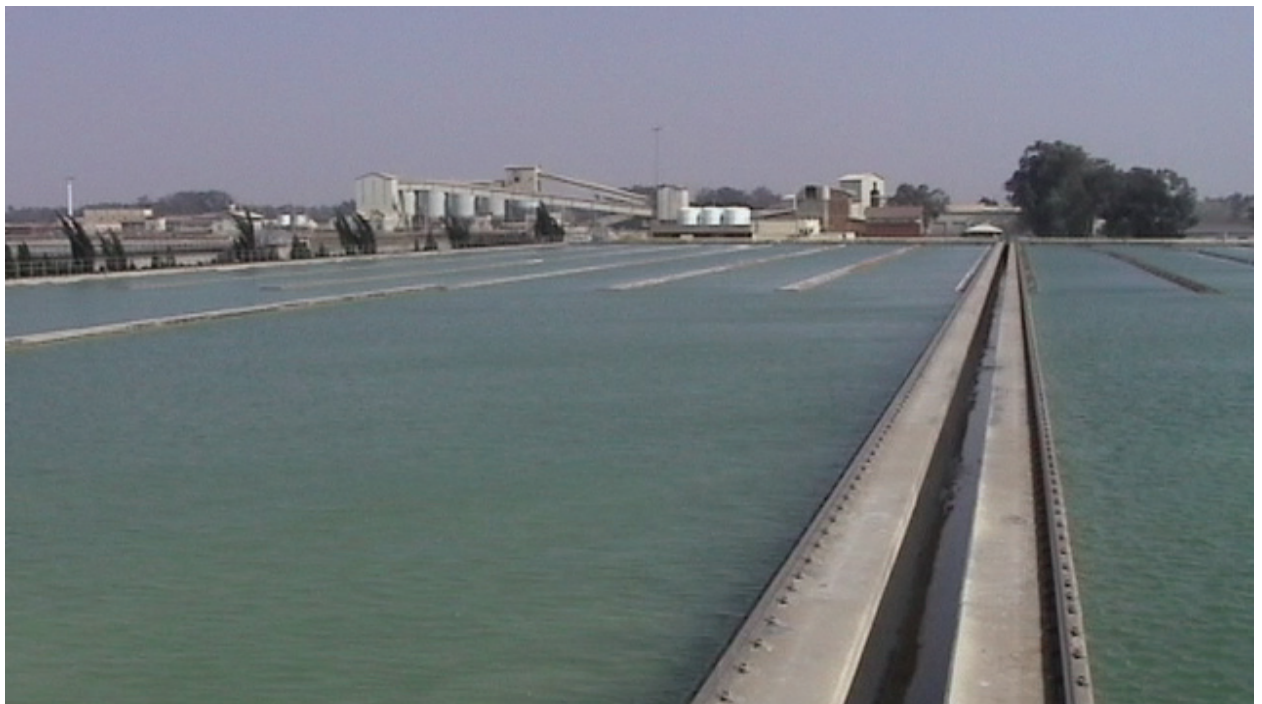
Figure B2.3: Horizontal sedimentation tank
